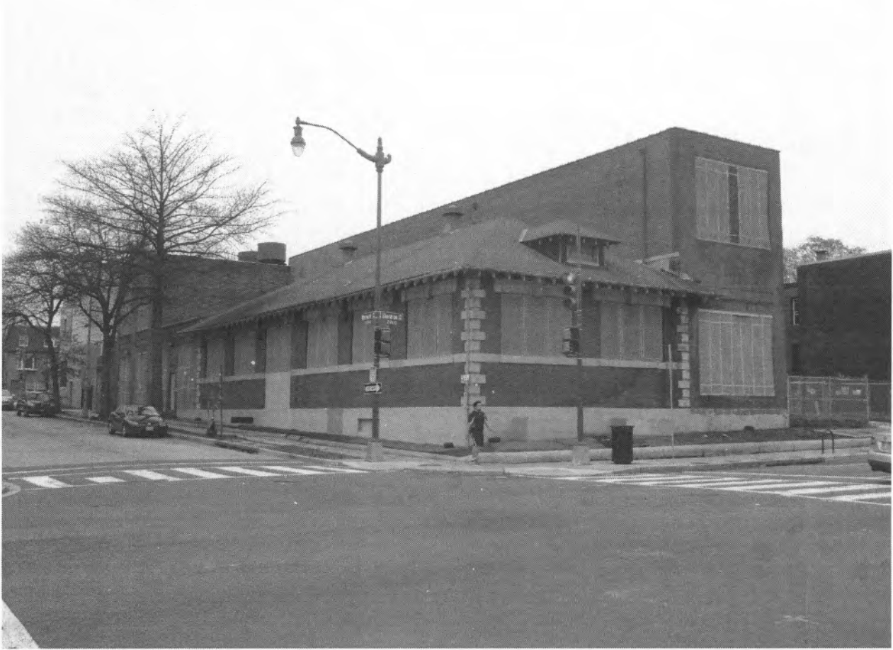
Pepco Substation No. 13
