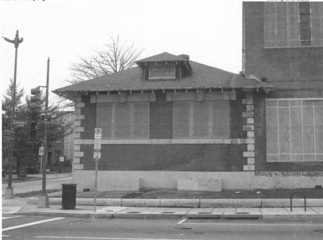
Pepco Substation No. 13
