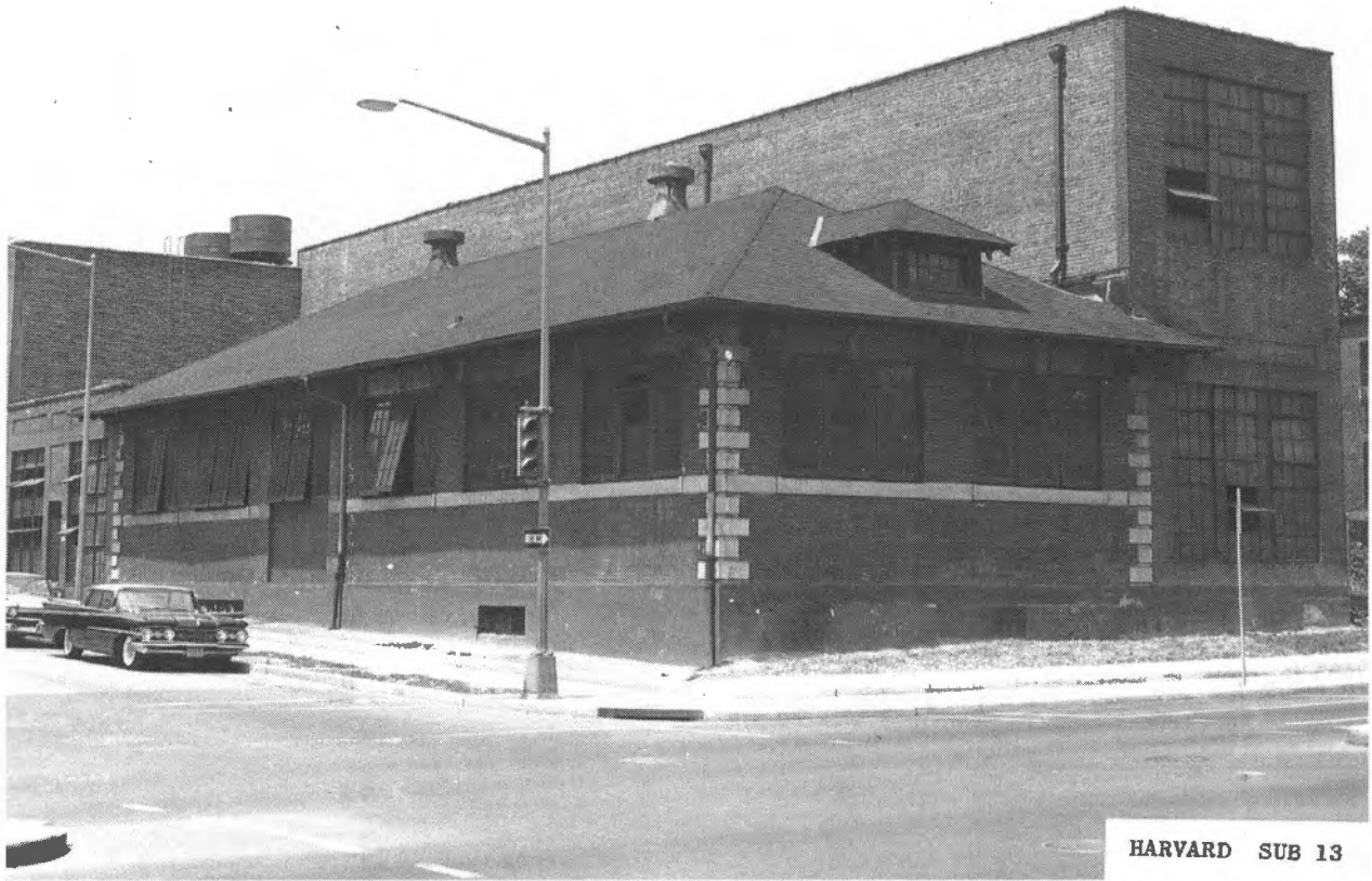
Potomac Electric Power Company Substation No. 13, view toward the northwest from the intersection of Sherman Avenue and Harvard Street, NW, ca. 1950s. (Photo from Pepco)
