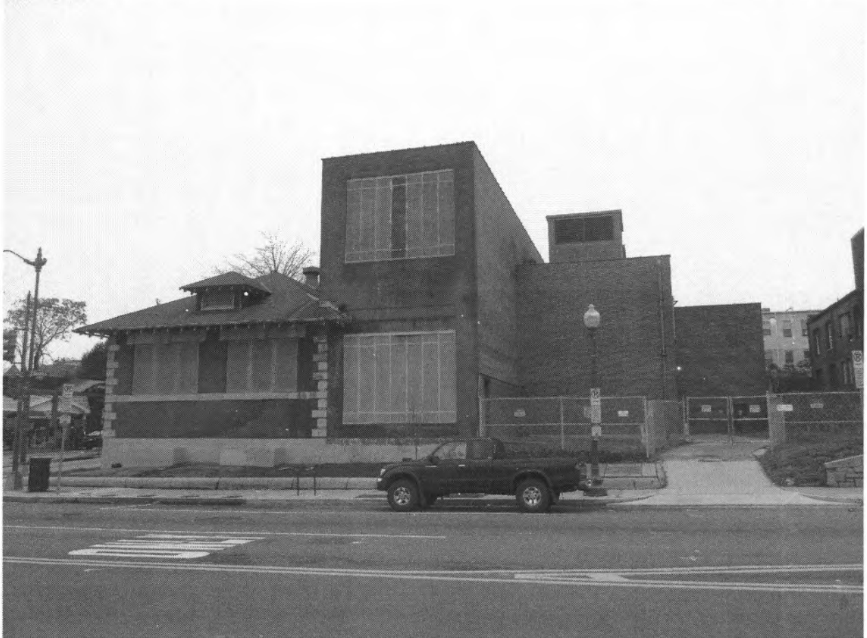
Pepco Substation No. 13
