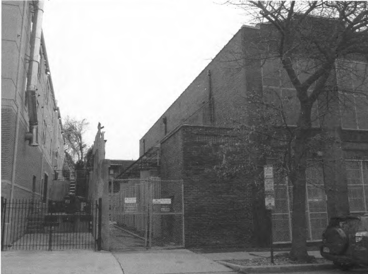
Pepco Substation No. 13
